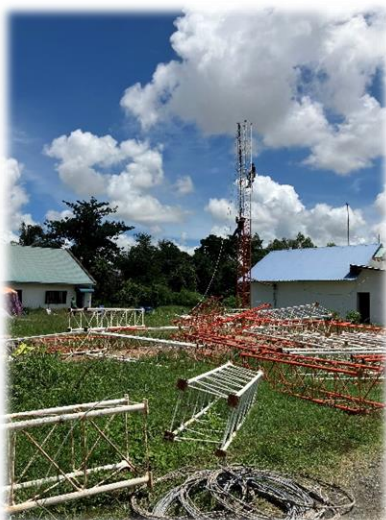
DISMANTLING THE OLD TOWER
